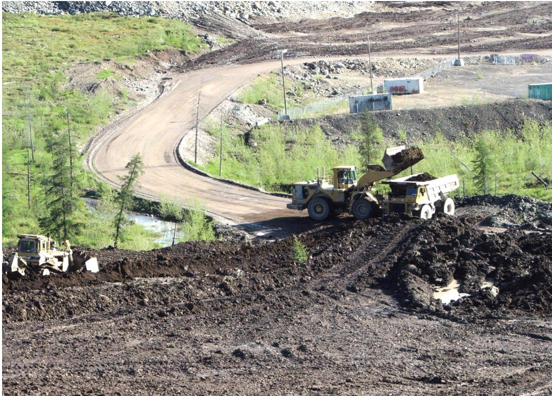
Figure 2. Using of soils reserve from native communities for formation root layer on rock dumps (Gold mine Kubaka in Kolyma river basin).
