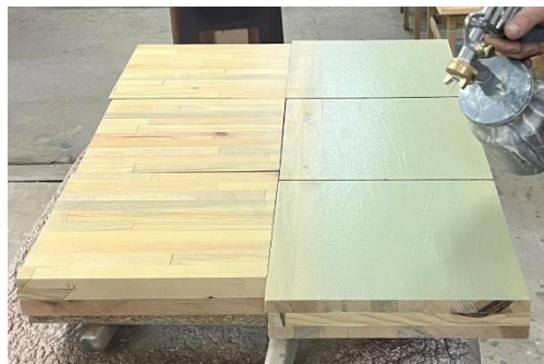
Figure 4. Application of thermal insulation paint.
