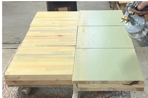
Figure 4. Application of thermal insulation paint.
